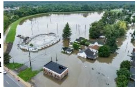
This aerial photo shows some of the flooded area in Anderson.
