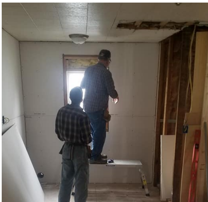
All new drywall was hung.
