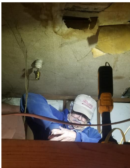
All the wiring had to be replaced.
