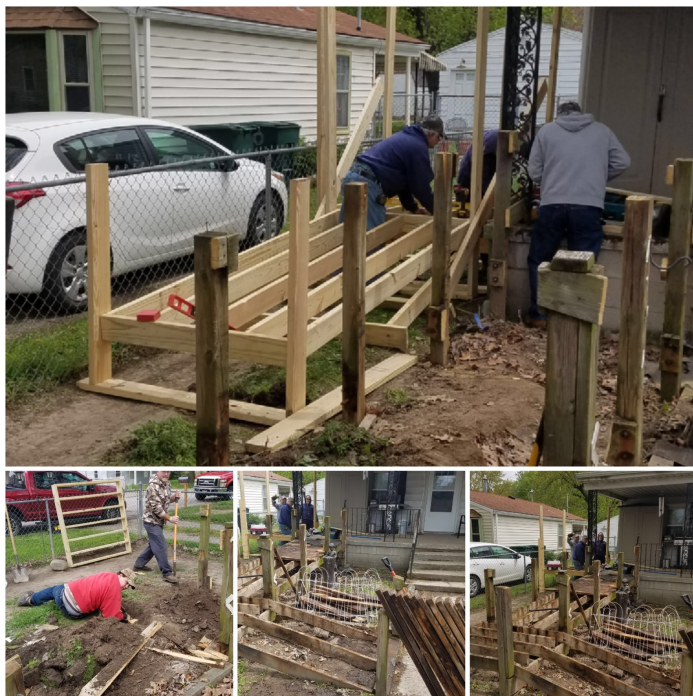
Disaster Relief Team works on building a wheelchair ramp.
