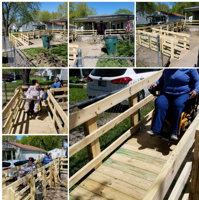
Completed ramp is a joy for the family.
