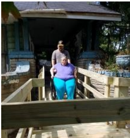
The first time out of her house in 1 1/2 years, thanks to the wheelchair ramp built by DR
