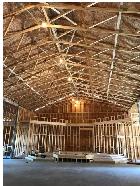
Sanctuary under construction inside.
