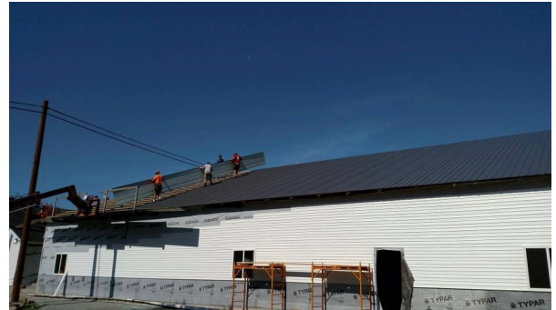
Putting on the metal roof of the new sanctuary at New Day Baptist Church in Alexandria.
